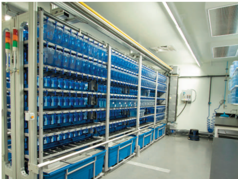
Modern zebrafish facility with focused lighting and Tritone automated feeder. Note the focused lighting over the bench tops. Image: Erik Sanders.
