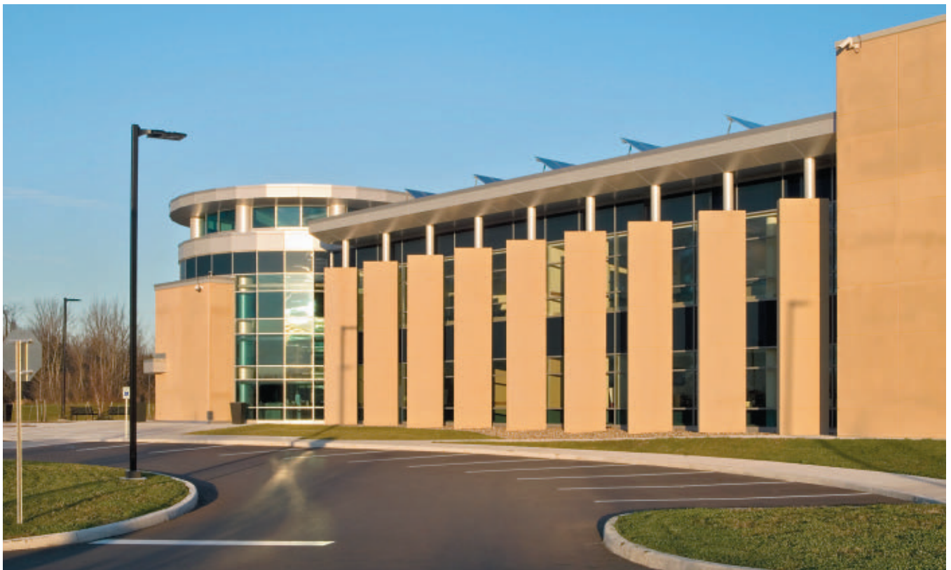
Evaluation of the building envelope, including existing energy features such as solar shades and photovoltaic panels, constitutes a major component of a Comprehensive Energy Management plan. All images: Randall Perry; Courtesy of SMRT Architects and Engineers.
